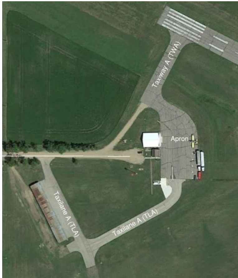
Figure 4-22: Terminal Area, prior to 2019 Apron Project
